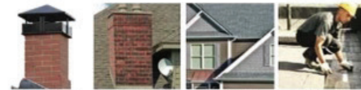
CHIMNEY LINERS CHIMNEY REPAIR CHIMNEY REPAIR CHIMNEY REPAIR
