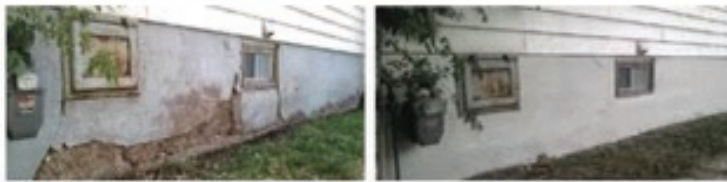
FOUNDATION REPAIRS BEFORE & AFTER
